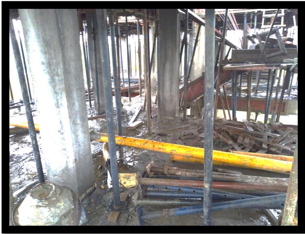
Block -1 (1BK type) structure 2 nd Floor Level
