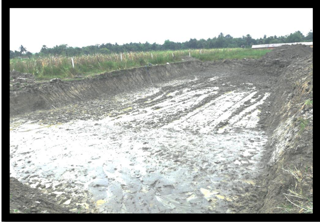
Block - 18 & 19 (2BHK type) foundation excavation completed
