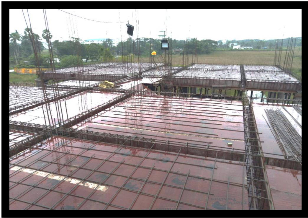
Block-1 (1BK type) 3 rd Floor level structure work ongoing
