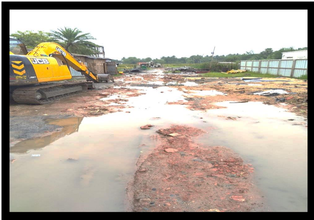
Project road filling completed
